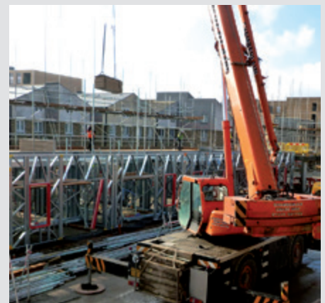
Crane lifting materials into position from agreed crane set area
