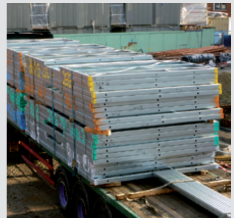
Delivery of wall panels on articulated vehicle with access to site
